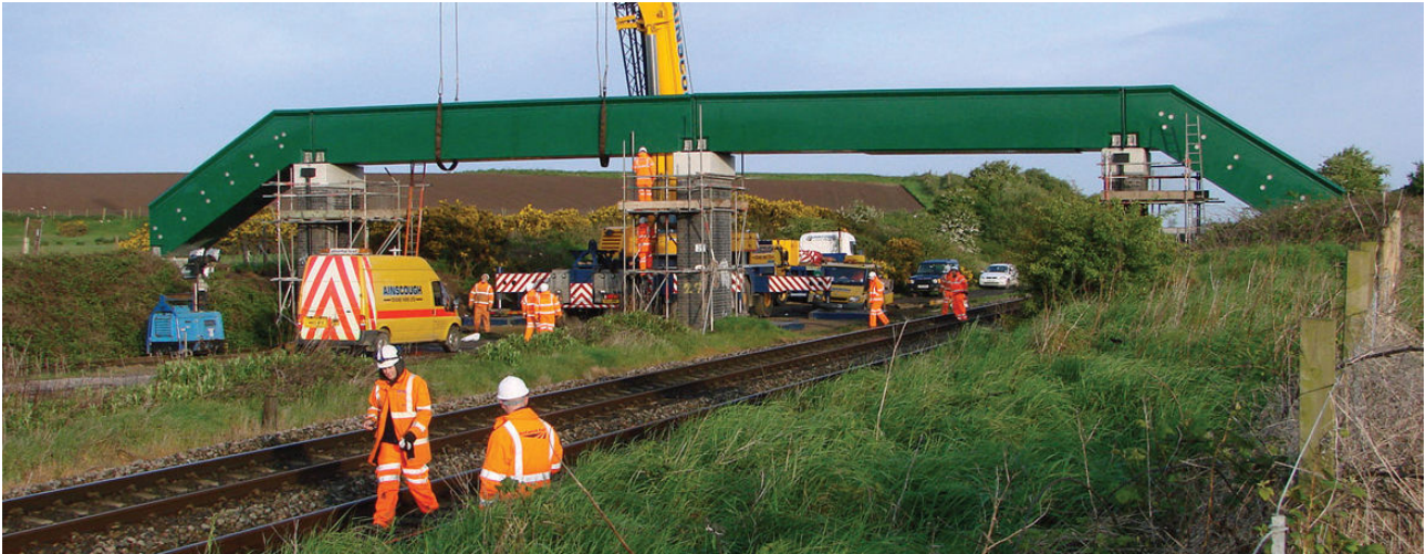
GRP Bridge constructed over railway line in slight cutting.
